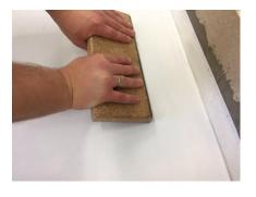
In the edge area adhere to the existing sealing tape. Adjoin seams of the sheets.
