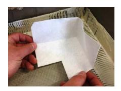
Mark corners, apply WAKOL MS 550 PVC and Rubber Adhesive, insert WAKOL AS 153 Sealing Corners, inner and grind..
