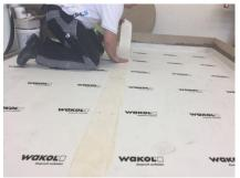
Coat the marked area on the left and right of the joint with WAKOL MS 550 PVC and Rubber Adhesive and wait at least 20 minutes.
